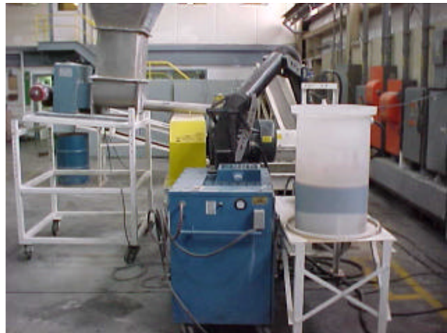
Photo 2 – Feeding and Binder Tank
